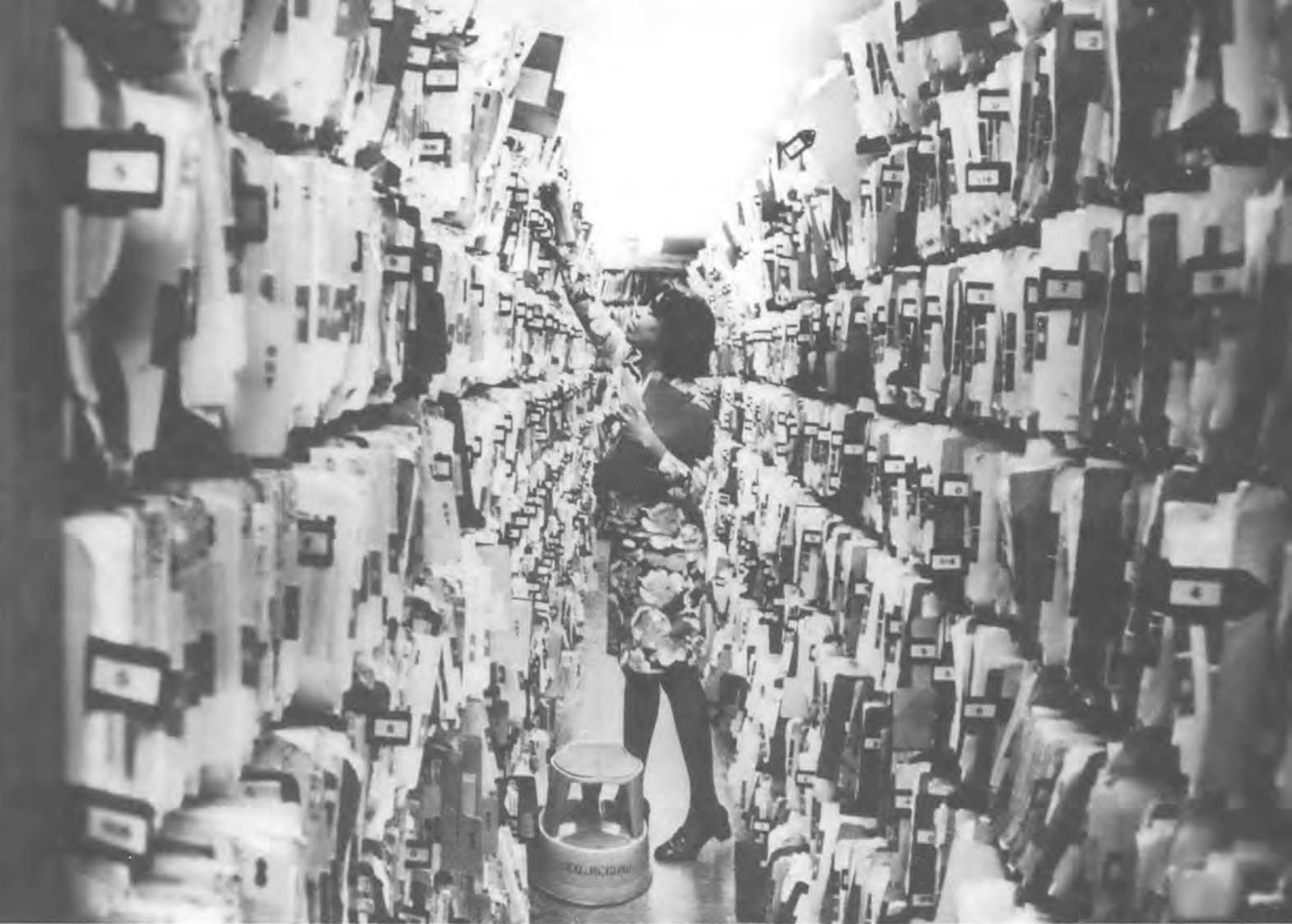
Several weeks after this photo was taken in a hospital basement, this entire wall of files collapsed. photo courtesy American Federation of State, County and Municipal Employees.
