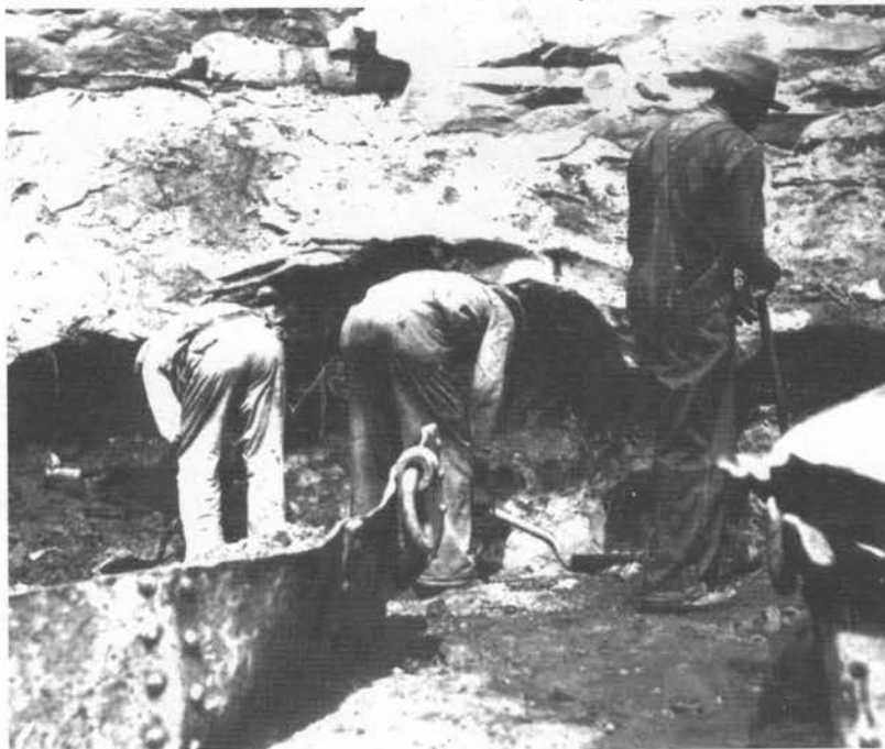
BLACK WORKERS DIG THROUGH DEADLY SILICA AT GAULEY BRIDGE, WEST VIRGINIA IN 1930.
