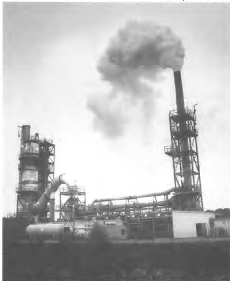
Superfund cleanup incinerator looms over Slidell, Louisiana.
