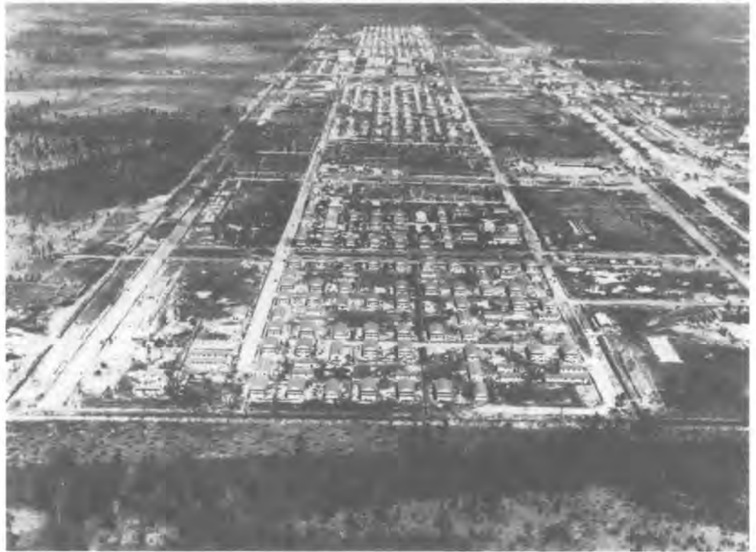
This aerial view of Camp Davis, North Carolina, shows the amount of construction just three months after it began in 1941.
