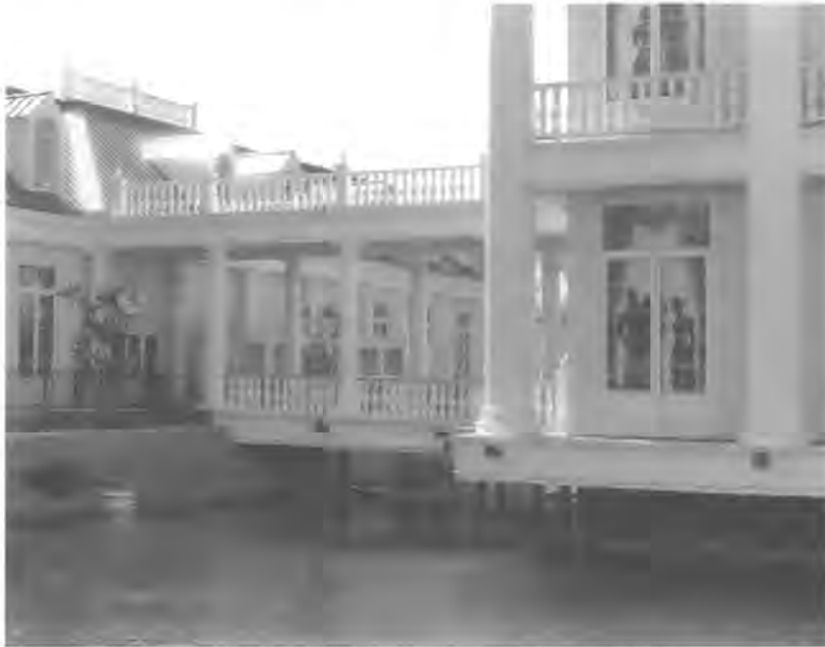
HARRAH'S AND MOST OF THE OTHER RIVERBOATS IN TUNICA ARE NOTHING MORE THAN PALATIAL STRUCTURES BUILT ATOP DOCKSIDE BARGES.
