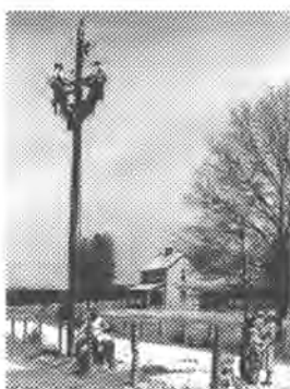
Photo courtesy of Tennessee Valley Authority
