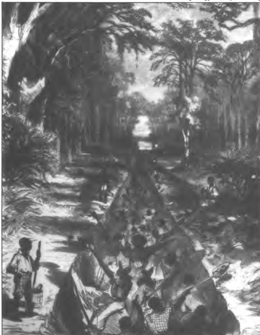
BLACKS DIGGING A CANAL NEAR VICKSBURG, MISSISSIPPI.
