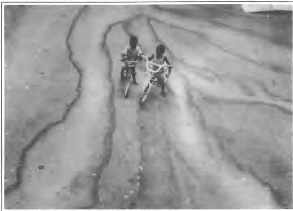
RAW SEWAGE STAINS THE PARKING LOT AT A HUD-SUBSIDIZED APARTMENT COMPLEX IN MIAMI.
