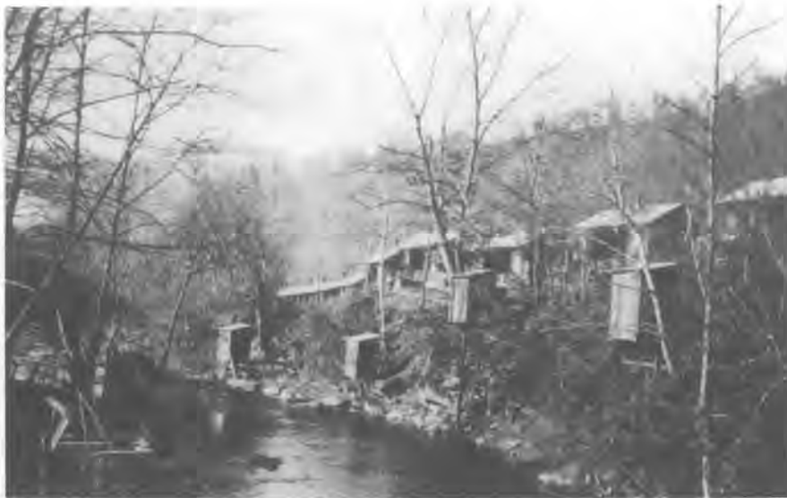
Privies at Proctor, North Carolina, showing how waste emptied directly into streams. This view is from a bridge on the main street of the small village.
