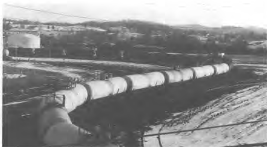
A moving pipe line carries unknown chemicals through the TEC complex.
