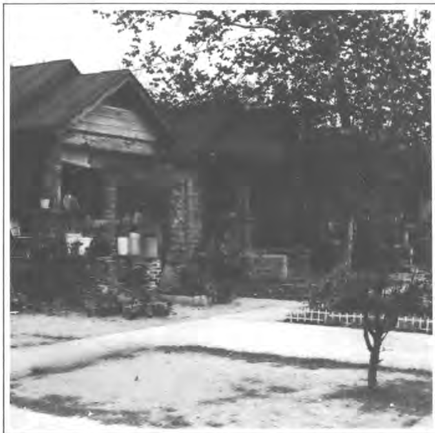
RAILROAD HOUSES IN NEED OF REHABILITATION
