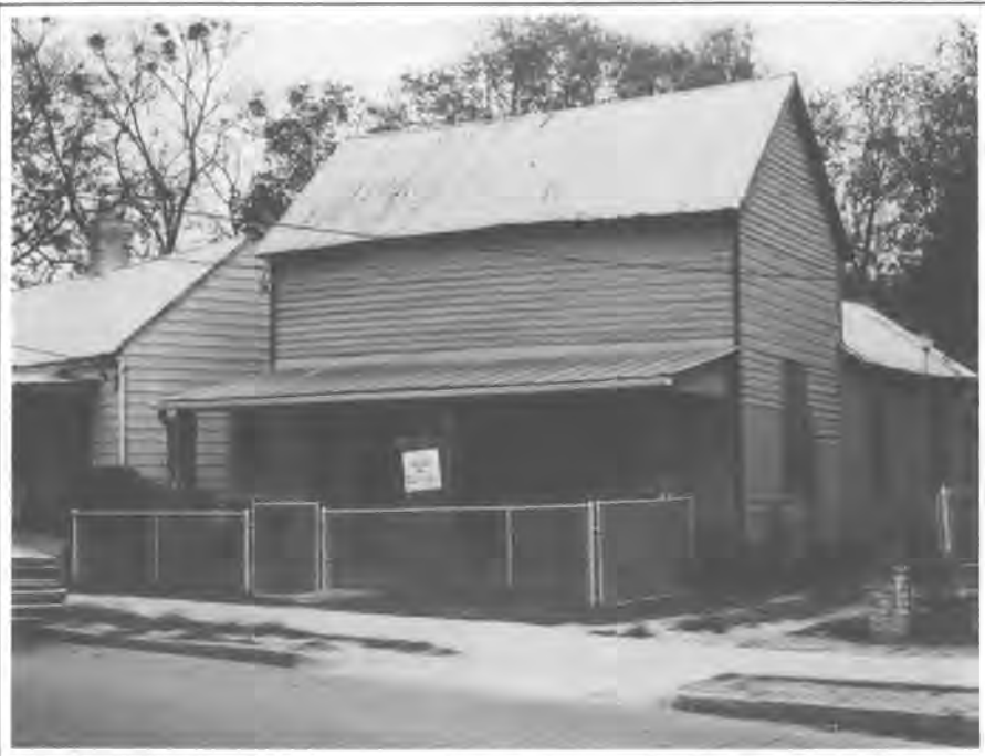
THE JOSHUA BONDS HOME, RESTORED BY BACA AS AN OFFICE AND COMMUNITY CENTER
