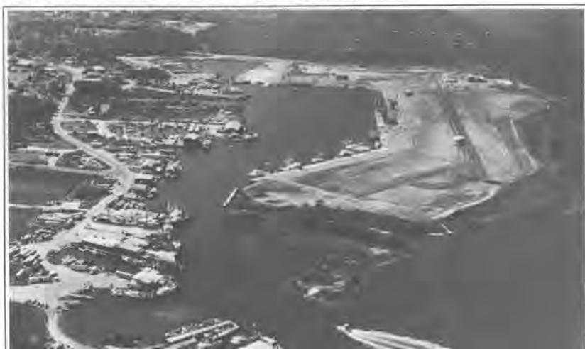
AN AERIAL VIEW OF THE SEAFOOD INDUSTRIAL PARK
