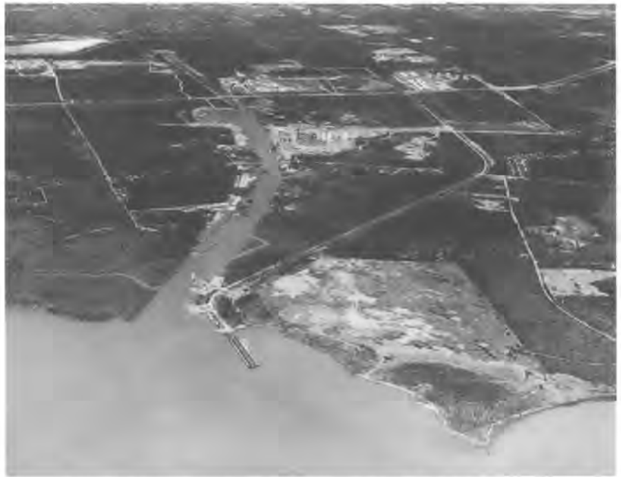
AERIAL VIEW OF THEODORE INDUSTRIAL PARK AND ITS WATERWAY
