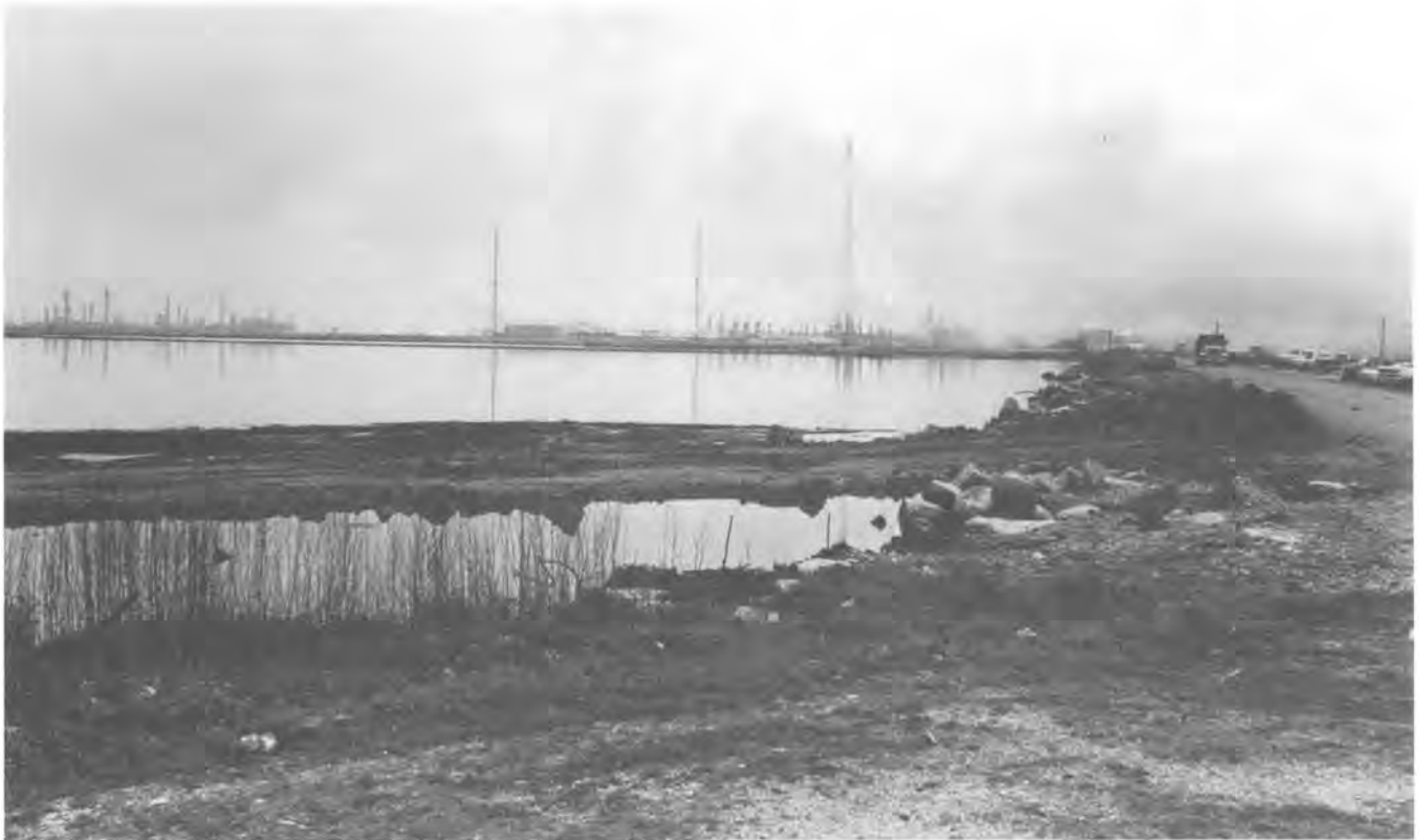
View of the Texaco refinery on the day of the explosion.
