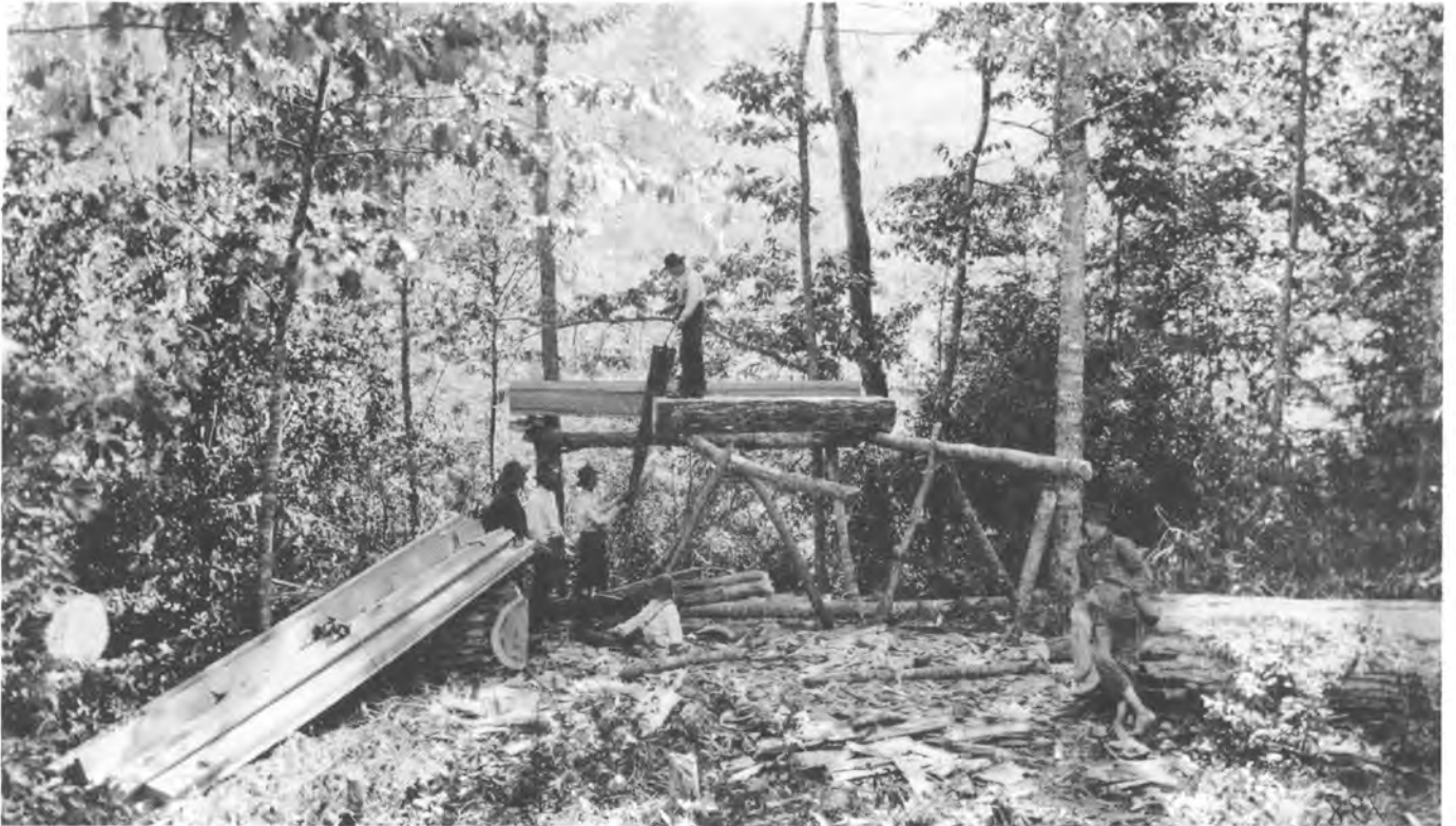
"Whip-sawing" near head of Browney's Creek, Harlan County, Kentucky, 1886.
