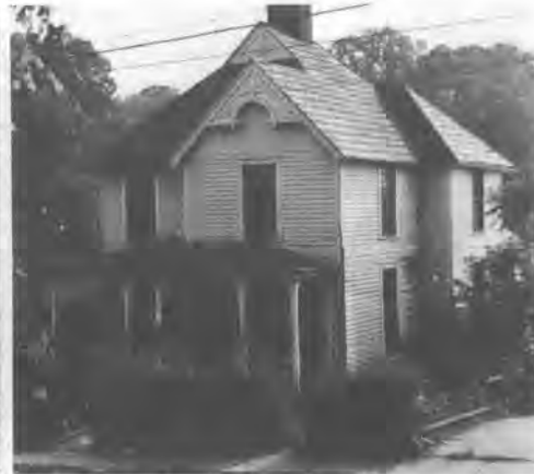
The house above, donated by a local business, will be moved to a vacant lot.
