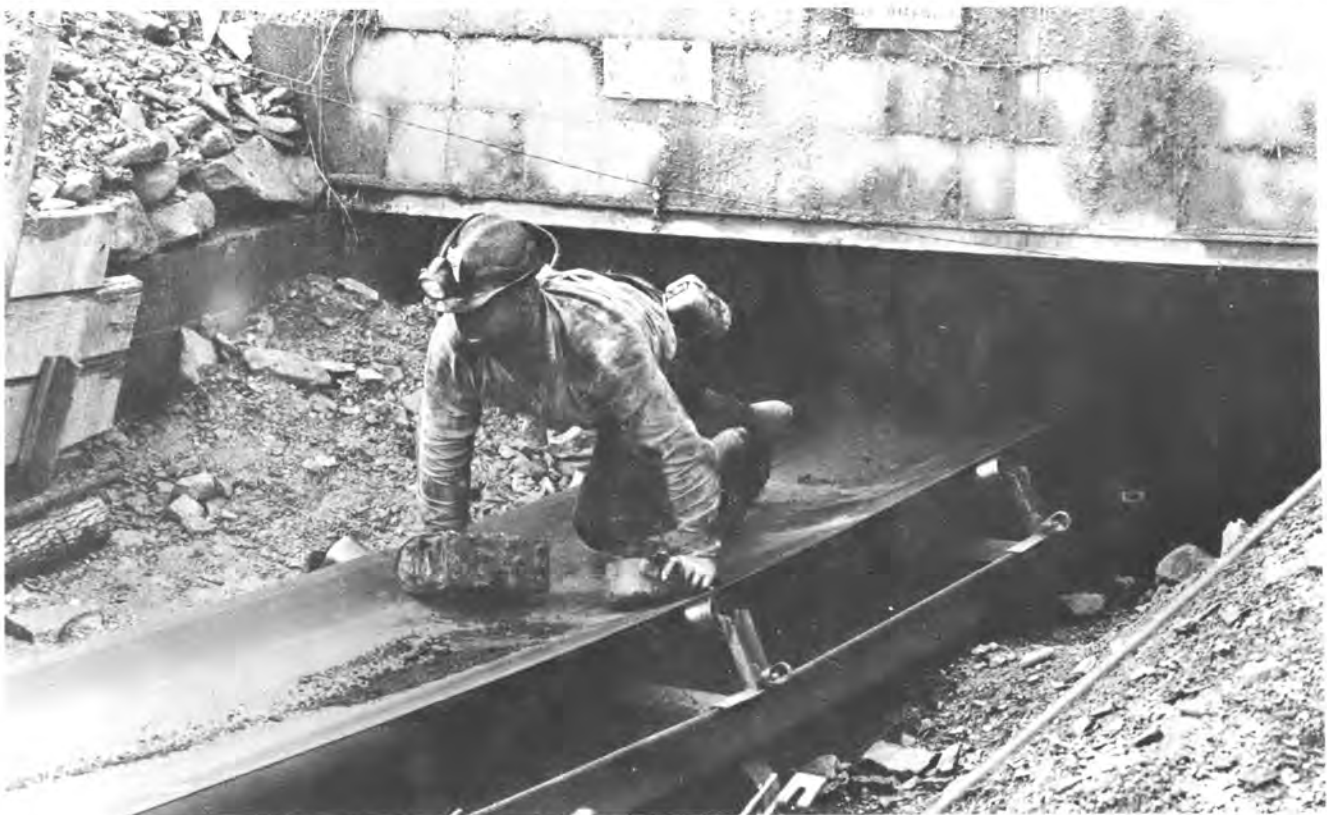
Riding the conveyor belt to and from the work area at an operating UMW mine.
