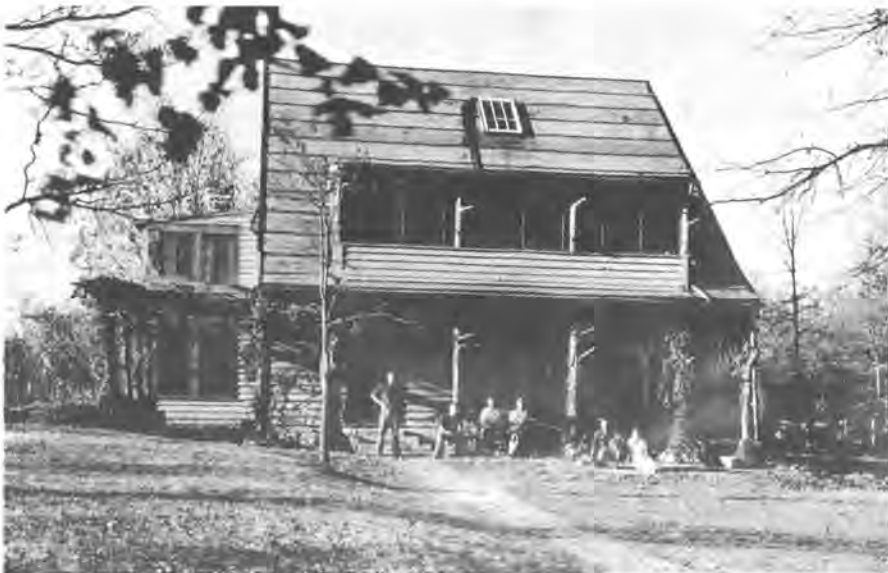
Front of main building of Highlander at Monteagle
